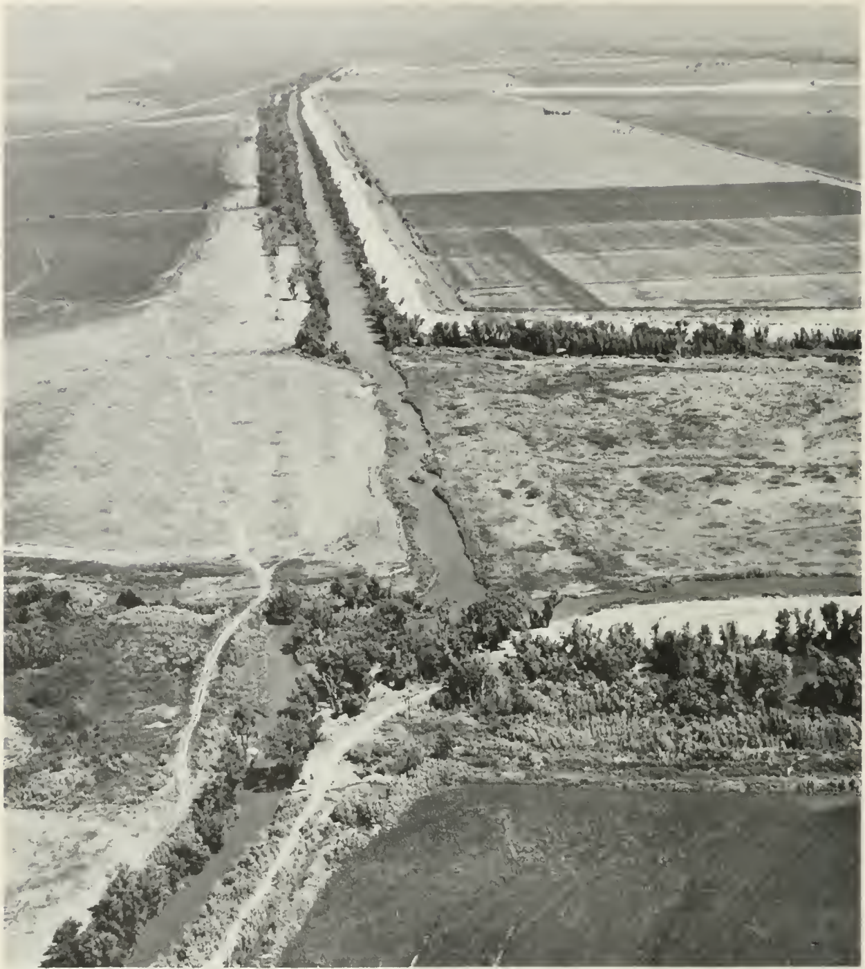
View of the Tule Canal looking northward showing Sacramento Bypass entering Yolo Bypass from the right side of photograph, and the much restricted channel of the Tule Canal.
