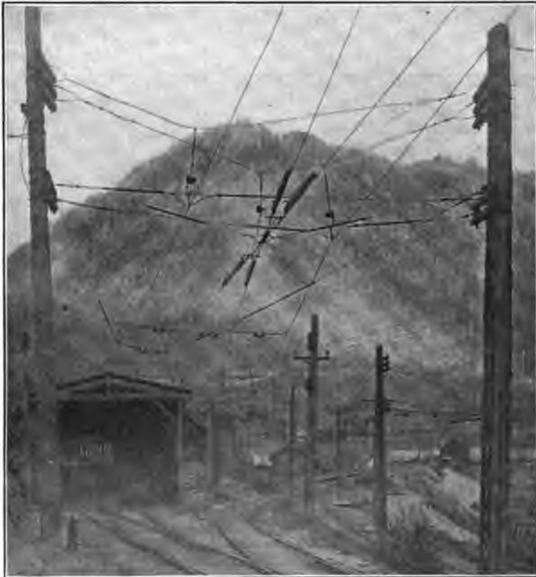
FIG. 15.—Construction at switch point, Wellington yard
