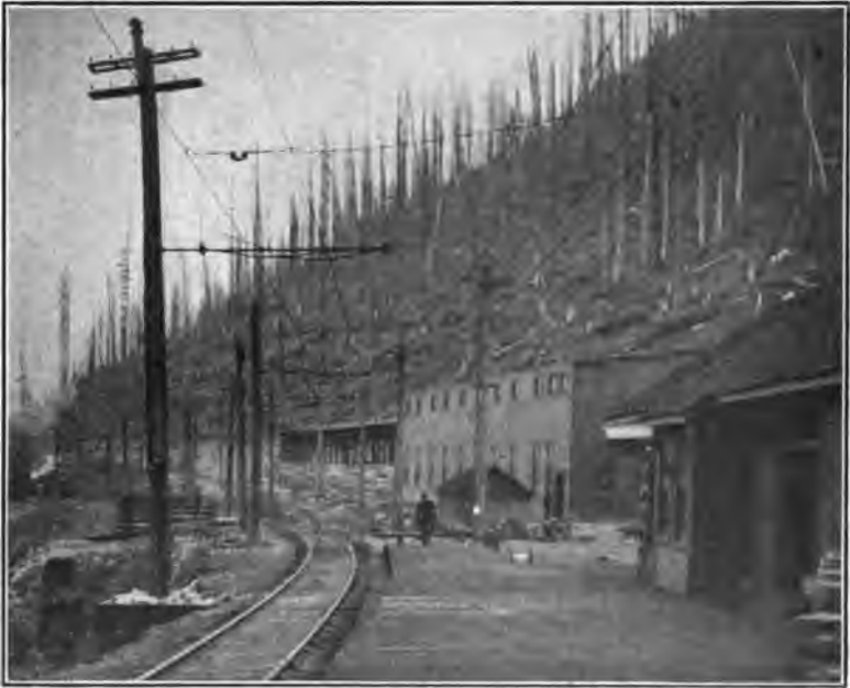
FIG. 16.—Bracket construction at curve Wellington yard
